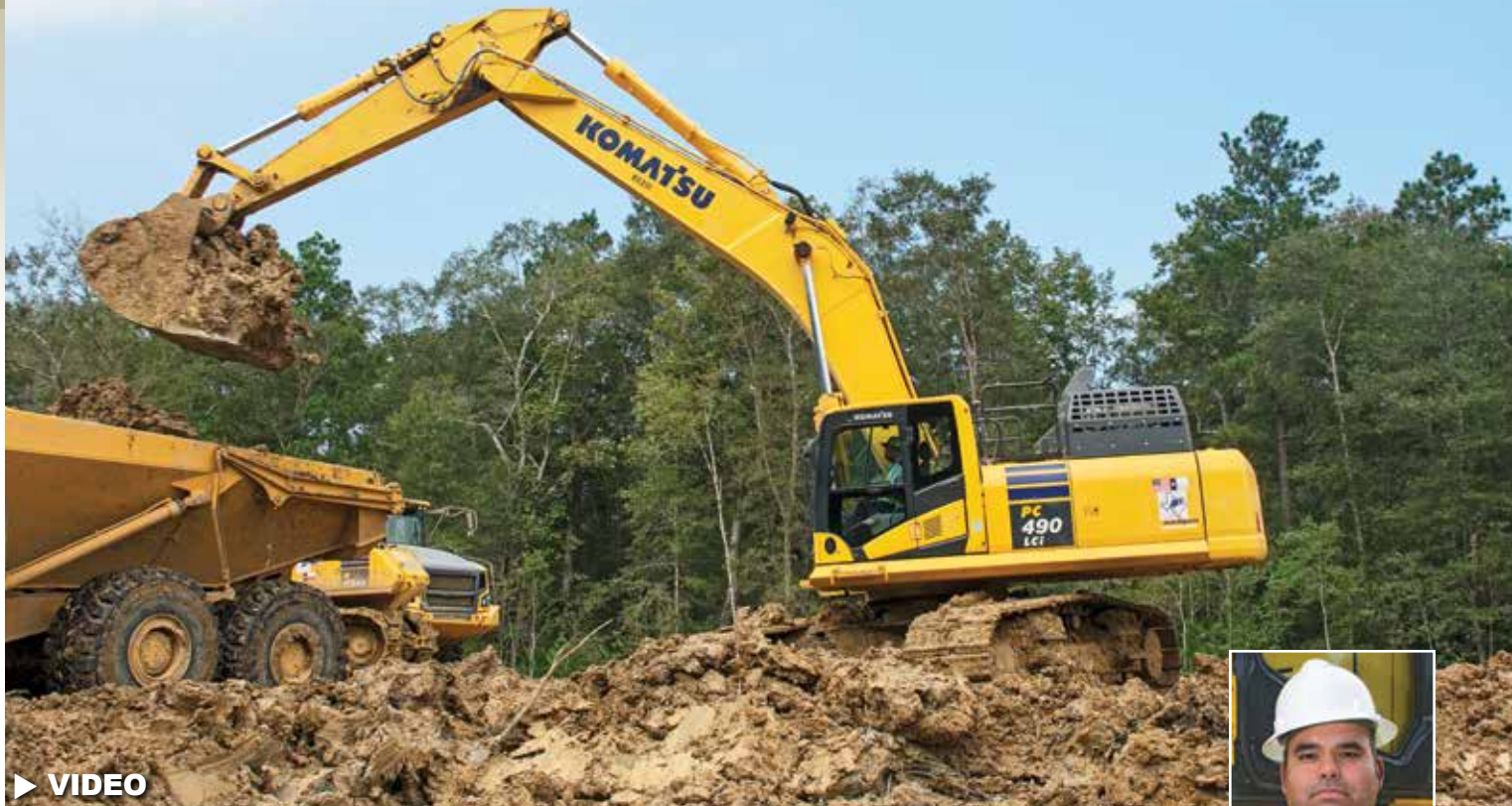
Operator Sergio Bellestros loads trucks with a Komatsu intelligent Machine Control PC490LCi on a canal project near Houston. "It's like a knife through butter," said Bellestros of digging with the excavator. "With the built-in GPS I can get to grade without worrying about overcutting or having to leave it a certain elevation for a dozer to finish."
